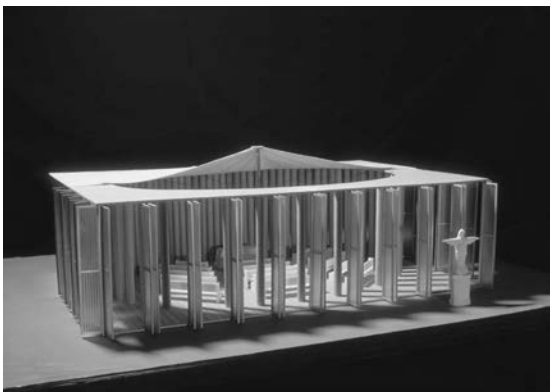
III. 5. Takatori Catholic Church/Paper Church, Kobe, 1995, architect: Shigeru Ban (structural system: 58 PTS (paper tube structures), partly steel frame)
