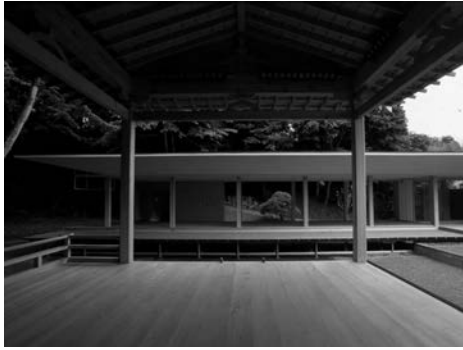
III. 6. Noh Stage in the Forest, Toyama City (Miyagi Pref.), 1996, architect: Kengo Kuma (structural system: cedar wood elements, reinforced concrete)
