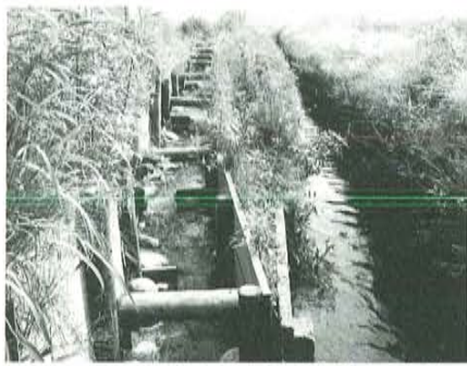
Fig.1 水田と排水路を結ぶ小型水田魚道 A fish ladder connecting a paddy plot and a drainage canal
